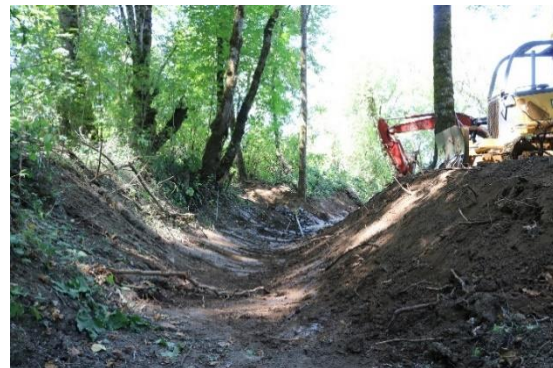
Reestablishing the oxbow connection to the Willamette River (before and after)
